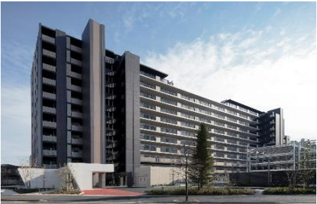
Kawagoe Nandai Rebuilding Project
