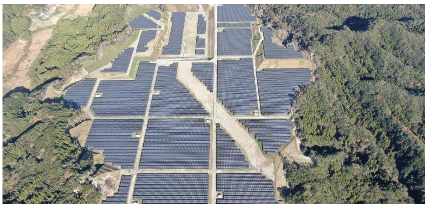
Leben Solar Chiba Katsuura power generation facility, completed in 2021
