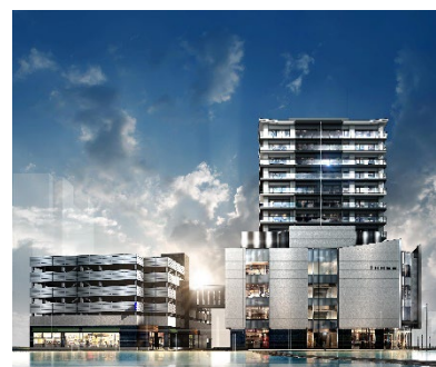
Project for Improvement of Excellent Buildings, etc. in the Shinmachi 1-chome Area
