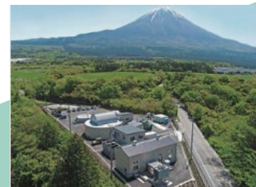
Fujisan Asagiri Biomass Power Plant
