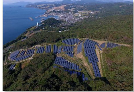
LS Nagasaki Isahaya power generation facility
