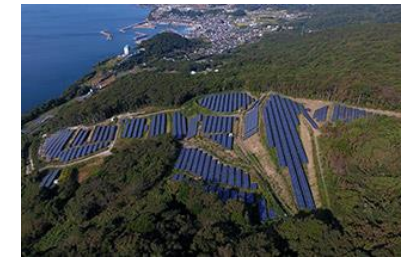
LS Nagasaki Isahaya power generation facility
