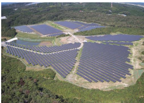
LS MIYAGI MATSUSHIMA power generation facility
