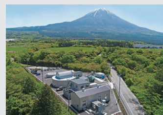
Fujisan Asagiri Biomass Power Plant
