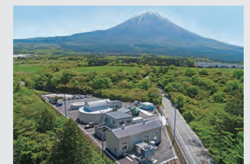
Fujisan Asagiri Biomass Power Plant
