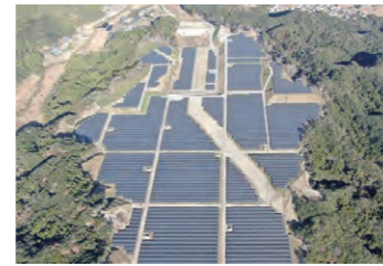
LS Chiba Katsuura Power Generation Facility
