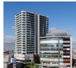
Minamikoiva 6-chome District Type 1 Urban Redevelopment Project
