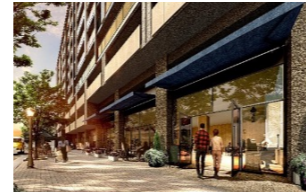
Urban Redevelopment of Machikatamachi and Toriyokocho District 1, Numazu City, Shizuoka Prefecture (conceptual image)
