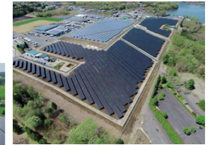
The LS Sakuragawa solar power-generation facility was completed in 2016.
