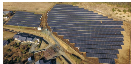
LS Takahagi Power Generation Facility
