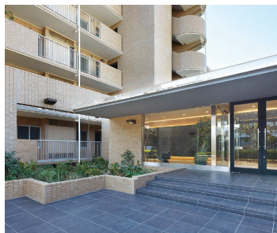
Le Art HIGASHI RINKAN THE RESIDENCE
