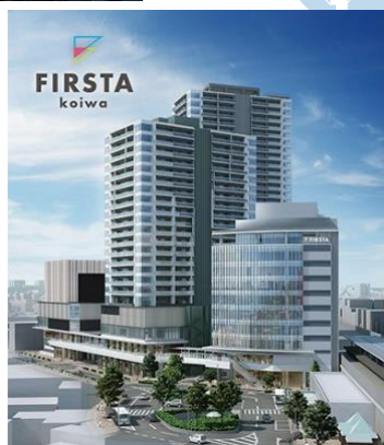
Minamikoiwa 6-chome Area Type 1 urban redevelopment project
