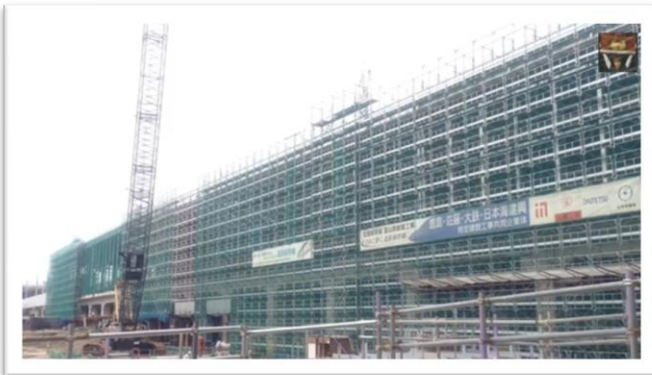
Construction of new Toyama Station building
