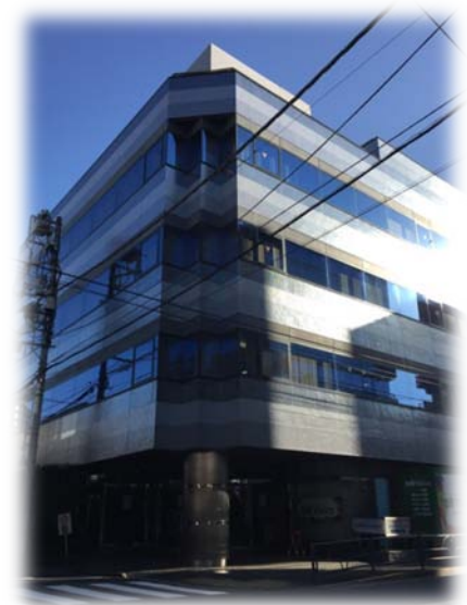
Nakano-daiichi OS building
