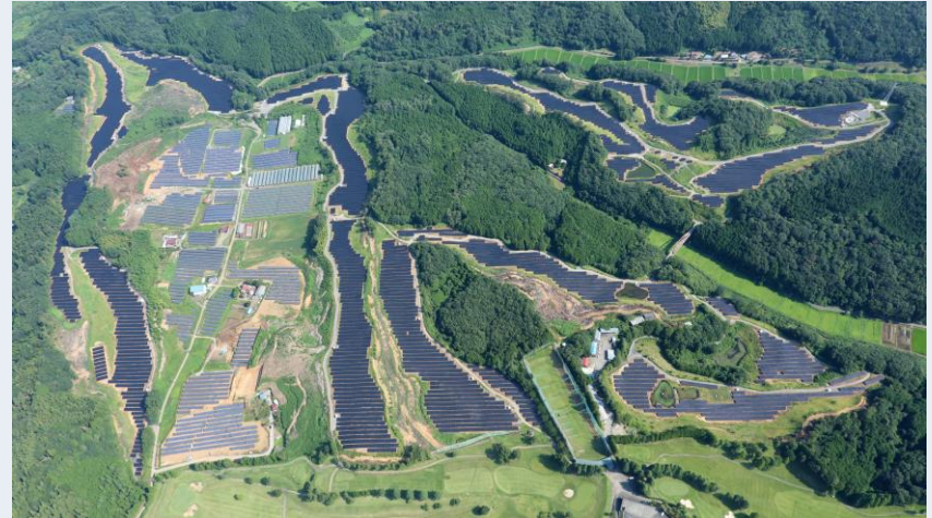
LS Nasu Nakagawa Power Plant
