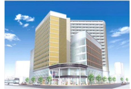
Sakura-machi, Toyama-shi Urban Redevelopment Project
