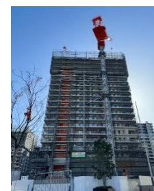
● Image at the time of construction
