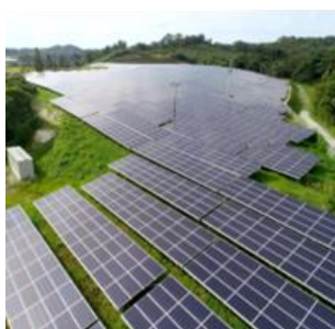
● Solar power plants
