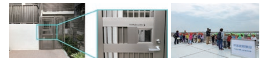
Entrance of emergency stairwell leading to the roof (1F, north side)
