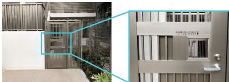
Entrance of emergency stairwell leading to the roof (1F, north side)
