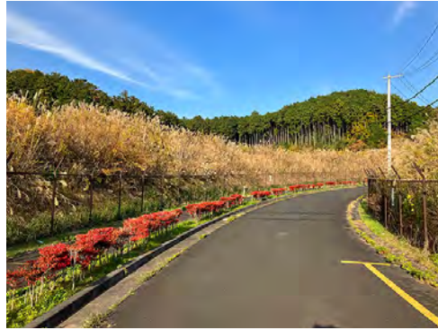
Roads around LS Hanno Misugidai Power Plant after weeding activities (Leben Community)
