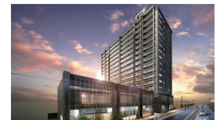
Case Takaoka City's lifestyle reinvigoration project for the western area of Suehiro LEBEN Takaoka MID RISE TOWER
