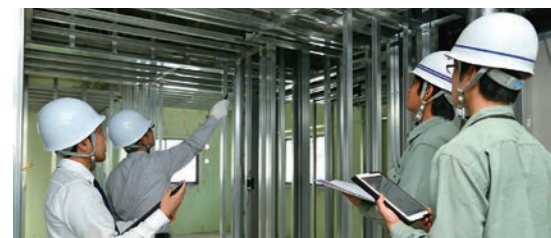
Site management during construction stage
